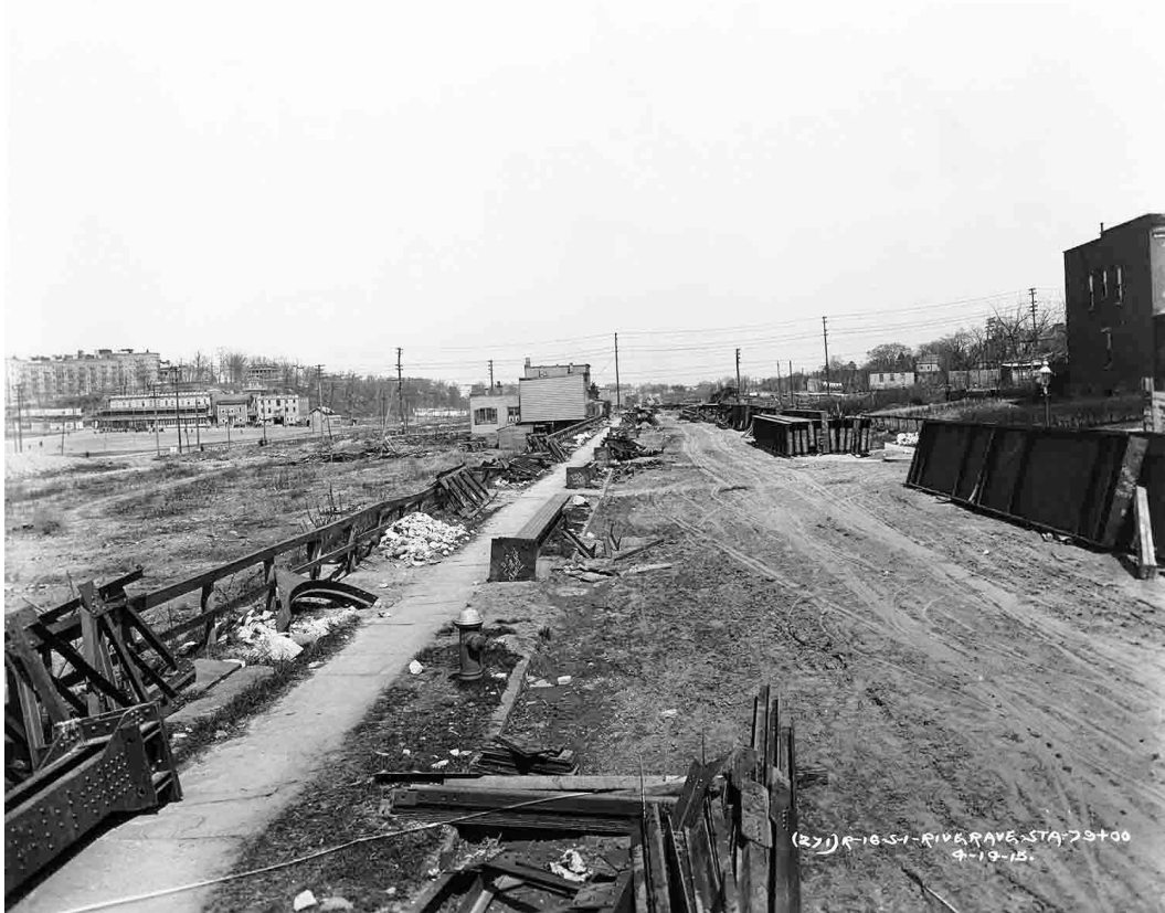
(Above and below) It is now April 14, 1915. The upper view is almost the same as the one on page 20, only this was taken a little east of River Avenue. The steelwork is being erected from the end of the ramp from the subway in a northerly direction. In the lower view, the photographer has walked to between 157th and 158th Streets and we see the steelwork stored on either side of River Avenue, waiting to be installed. Seven years and one month after this picture was taken, ground will be broken in the open field to the left for the first Yankee Stadium. Charles Manchester/PSC photo
