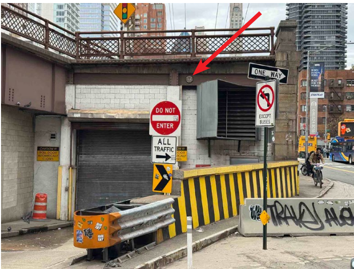
In this view taken on March 27, the railway plaque can be seen just to the right near the top of the center upright girder. Paul Grether photo
