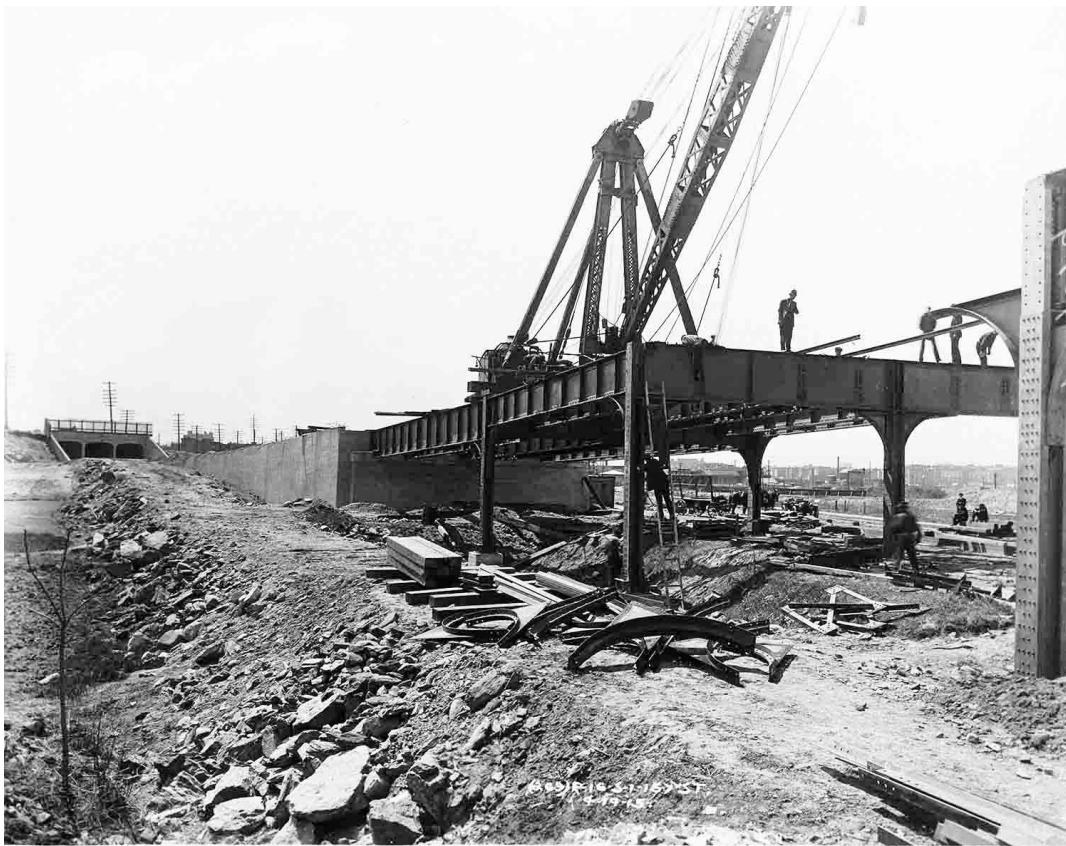
(Above and below) It is now April 14, 1915. The upper view is almost the same as the one on page 20, only this was taken a little east of River Avenue. The steelwork is being erected from the end of the ramp from the subway in a northerly direction. In the lower view, the photographer has walked to between 157th and 158th Streets and we see the steelwork stored on either side of River Avenue, waiting to be installed. Seven years and one month after this picture was taken, ground will be broken in the open field to the left for the first Yankee Stadium. Charles Manchester/PSC photo
