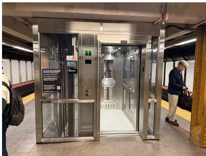
Elevator EL218, seen at platform level of the BMT Canarsie Line. Michael Cortez/MTA photo
