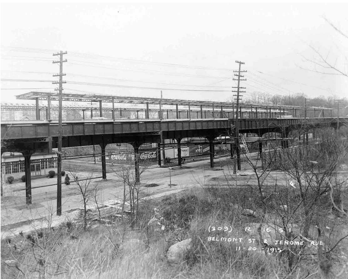
Continuing with November 20, we are 100 feet east of the east curb of Jerome Avenue, looking northwest at Belmont Street (now Mount Eden Avenue) Station. Charles Manchester/PSC photo
