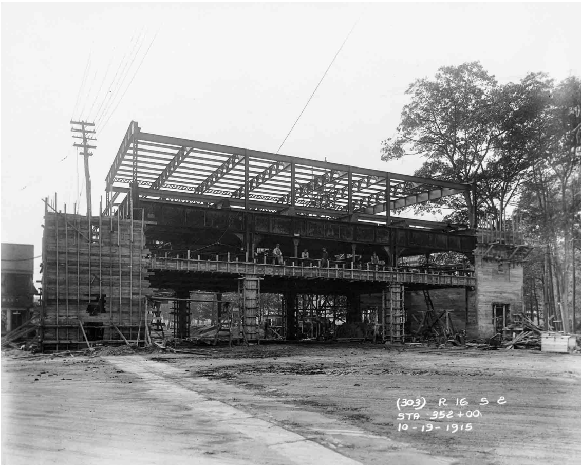
The same day as in the previous two images, this is looking southwest at the terminal station, Woodlawn, from the east building line of Jerome Avenue, at Bainbridge Avenue. Charles Manchester/PSC photo
