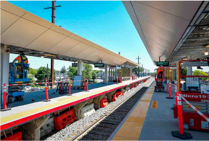
View east of the current situation at Babylon, with both platforms restored to their 12-car lengths. Marc A. Hermann/MTA photo
