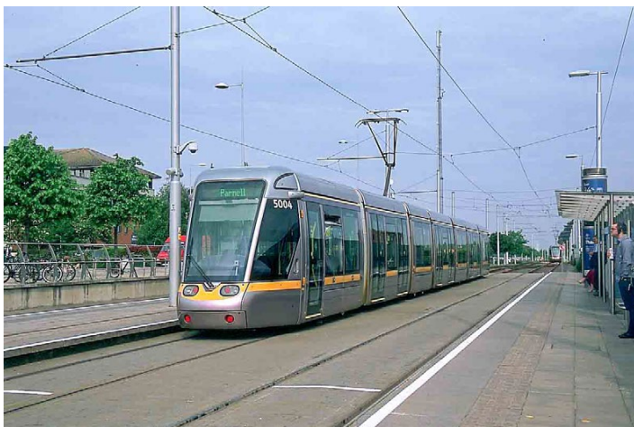
An Alstom Citadis 401 lays over as the Brides Glen terminal of the Green Line. It will loop at the Parnell stop at the northern edge of Dublin's business district. Service beyond Parnell is provided by cars that start at Sandford.
