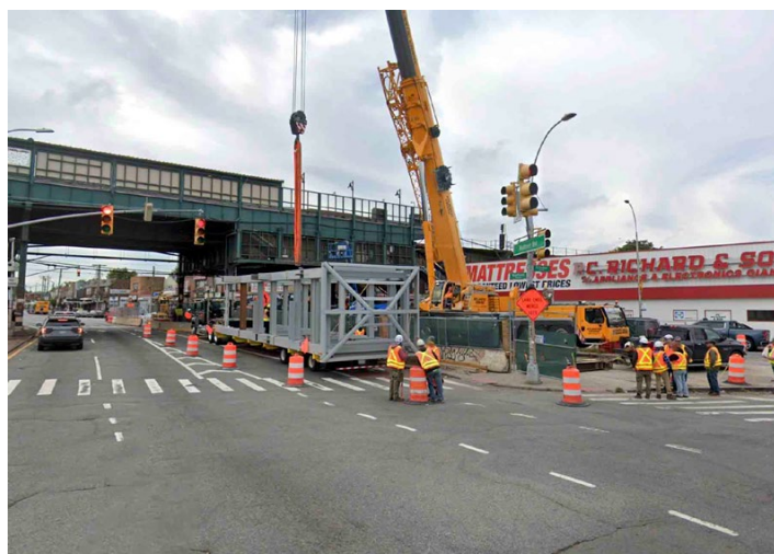
View south at Rockaway and Woodhaven Boulevards back in October 2024 showing the steelwork for the elevator that was going to be installed to the northbound platform. Google Street View photo
