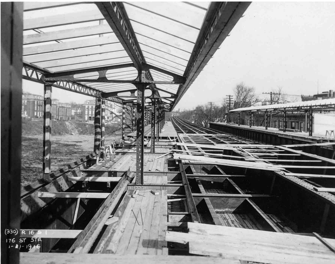
Same date as above. We are looking due north-northeast along the southbound platform at 176th Street Station. The steelwork completed, all of the woodwork is now being installed. This includes the platforms, windscreens and windows, canopies and the walls and rooms of the mezzanine. Charles Manchester/PSC photo
