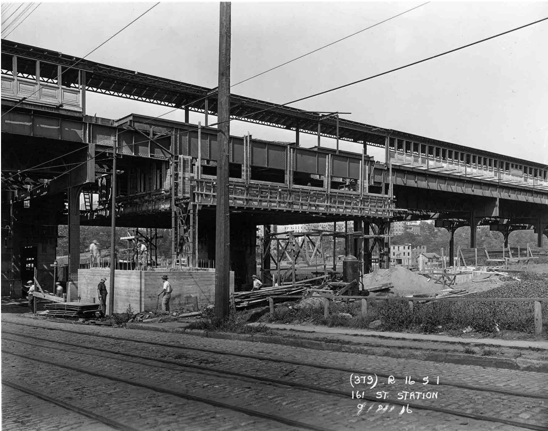
On the east side of the structure, the concrete work around the street stairs has not progressed as far. Looking northwest from the south curb of 161st Street.
