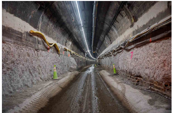
(Above and below) Two views of ERT Line 2 before the reconstruction started and during the benchwall demolition phase. Amtrak photos
