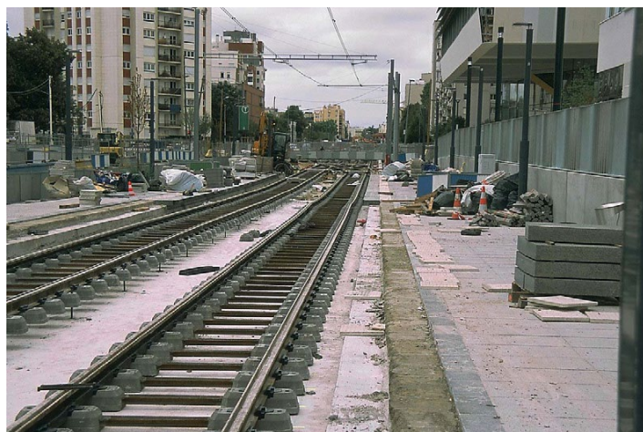
Looking east toward what was the temporary end of the line at Porte de Chapelle, some three months before service was inaugurated on the extension of Line T3b to Porte d'Asniers. It appears the stop was relocated to this exact point.
